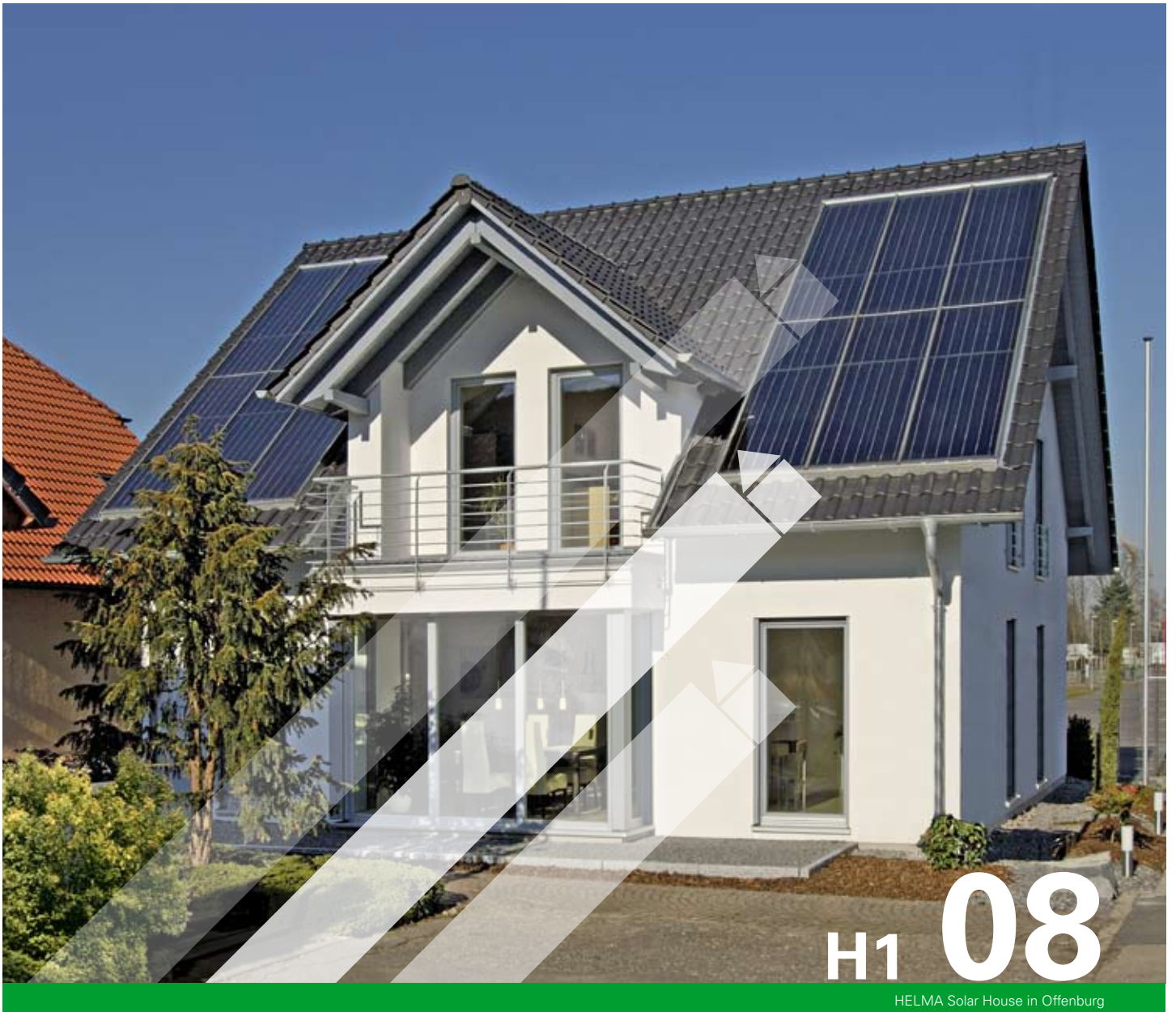
HELMA Solar House in Offenburg
